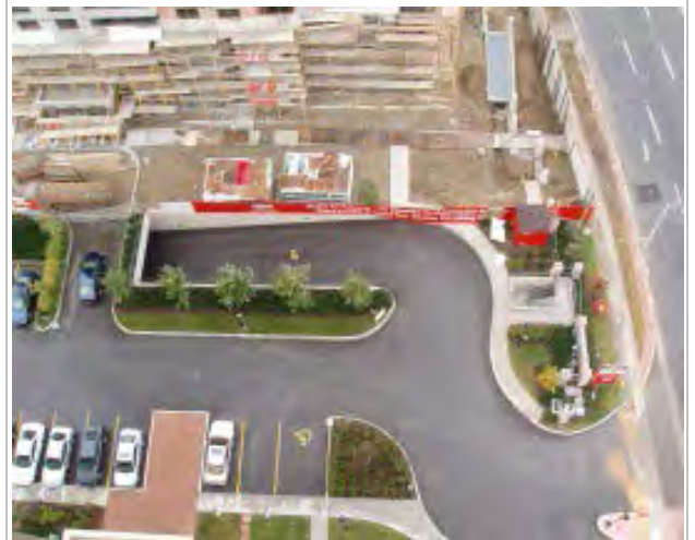
Essex 2 rising to the west As viewed from atop Essex 1 December 11, 2004
